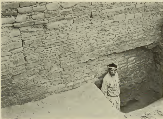
FIG. 163.—The overhang above the Indian's head shows the union of a new addition with older, partially razed walls in Pueblo Bonito. (Photograph by Neil M. Judd. Courtesy of the National Geographic Society.)
