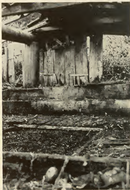
FIG. 180.—Interior of Eagle House. Two benches or floor levels rise on each side of the centrally excavated pit. The hearth is at the center of the pit, and the remainder of the floor including the two benches is covered with split cedar slabs. See figs. 177-179.
