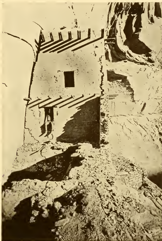
FIG. 119.—Tower from the west. New retaining wall at lower right-hand.
