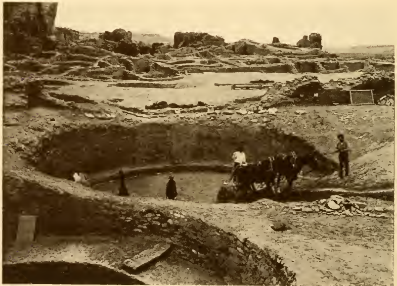
FIG. 100.—Excavating one of the major kivas of Pueblo Bonito. The flat roof of the subterranean room, 44 feet in diameter, had been supported by four wooden pillars. (Photograph by O. C. Havens. Courtesy of the National Geographic Society.)
