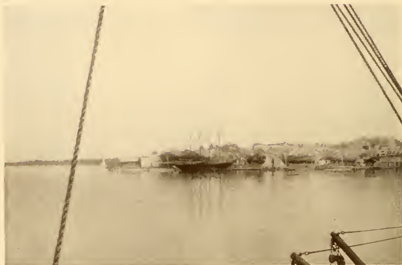
FIG. 48.—Pointe-a-Pitre, Guadeloupe. On account of quarantine regulations, no closer approach to the town was allowed during the winter of 1923-24.
