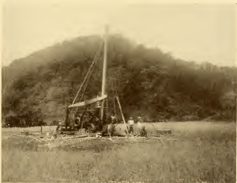
FIG. 25.—Drilling for oil, Neely's Fork, Clay County, Tennessee. (Photograph by Bassler.)
