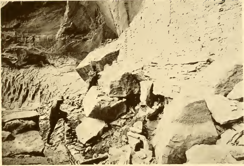
FIG. 120.—Looking west along the Tower at the beginning of repair.
