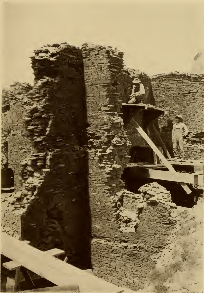
FIG. 116.—Repairing third-story walls in Pueblo Bonito. Some of these high walls had been so weakened by vandalism and the elements that their repair was necessary before excavation could safely be undertaken beneath. The work will serve, also, to preserve the present height of the walls for many years to come. (Photograph by O. C. Havens. Courtesy of the National Geographic Society.)
