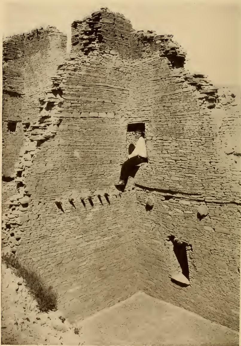
FIG. 117.—Repaired walls of the third type of masonry, showing occasional bands of thicker blocks inserted for strength and decorative effect. Corner doorways are not uncommon in Pueblo Bonito; they provided a direct means of communication between neighboring dwellings occupied by members of the same family or clan. (Photograph by Neil M. Judd. Courtesy of the National Geographic Society.)
