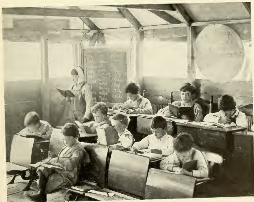
SEA BREEZE HOSPITAL, SEA GATE, NEW YORK. OPEN AIR SCHOOL Courtesy of Dr. J. W. Brannan
