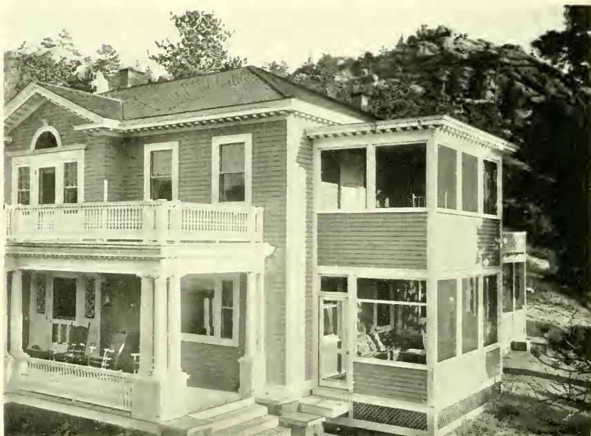
DOUBLE SLEEPING PORCH WITH EASTERN AND SOUTHERN EXPOSURES. THIS SUMMER RESIDENCE IN ESTES PARK, COLORADO, IS PROVIDED WITH PORCHES ON ALL SIDES SAVE THE NORTH, WHICH IS PROTECTED BY THE ROCKY FORMATION IN THE BACKGROUND. THE PORCH IS COVERED WITH A PERMANENT ROOF.
