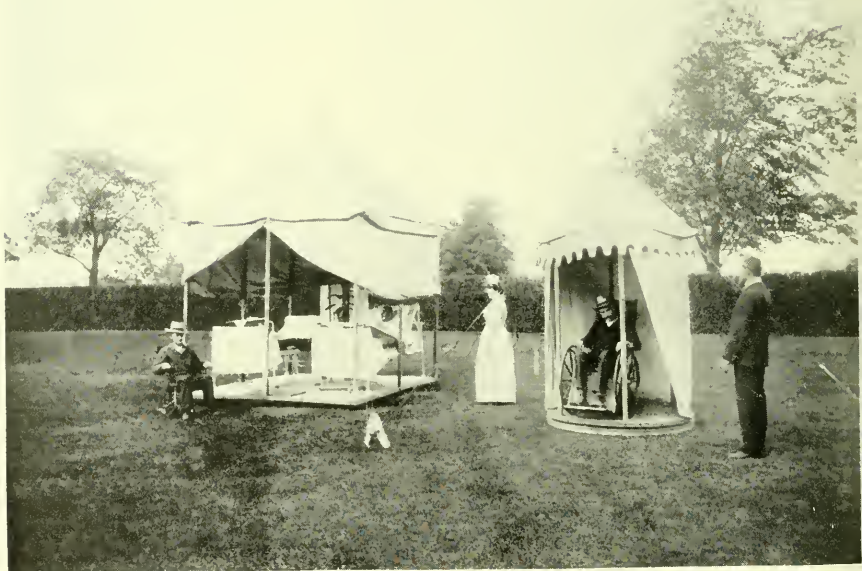
FIG. 2. MANHATTAN STATE HOSPITAL, EAST, CAMP A. INSANE TUBERCULOUS PATIENTS. REVOLVING TENT CONSTRUCTED SO AS TO BE EASILY TURNED IN ACCORDANCE WITH THE DIRECTION OF SUN AND WIND.
