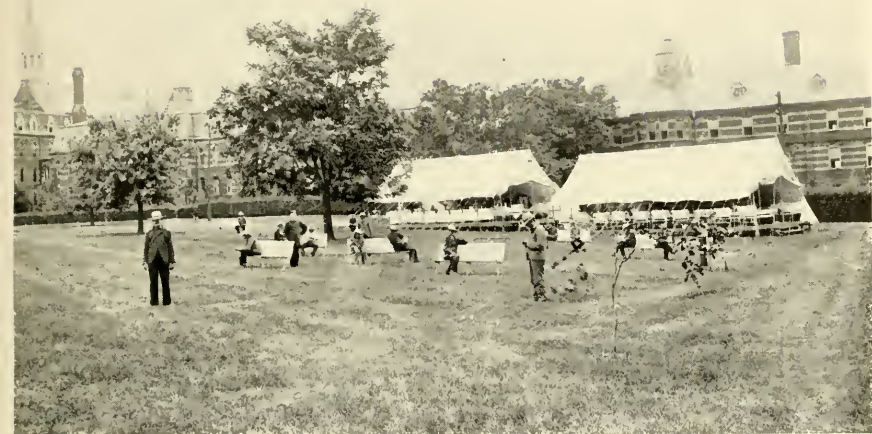
FIG. 1. MANHATTAN STATE HOSPITAL, EAST, WARD'S ISLAND, NEW YORK CITY. TENTS FOR THE TUBERCULOUS INSANE. SUMMER LOCATION
