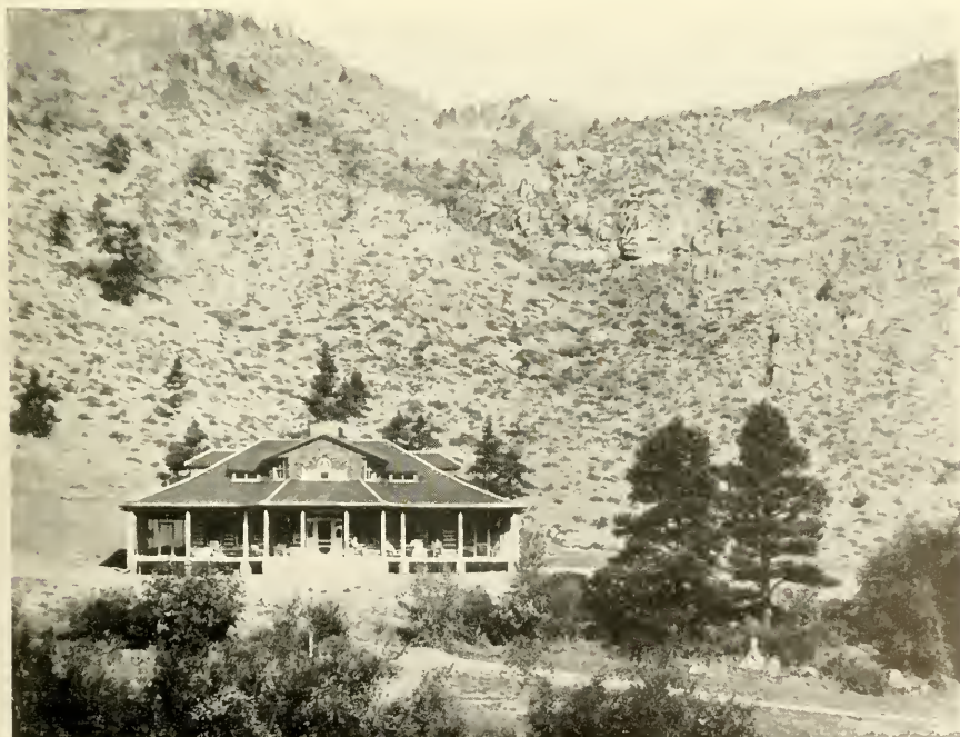
FIG. 2. ESTES PARK, COLORADO. IDEAL SUMMER RESIDENCE, WITH SPACIOUS PORCHES FOR PULMONARY INVALIDS. SLOPING GROUND, SANDY SOIL, MOUNTAINOUS BACK-GROUND AFFORDING PROTECTION FROM WIND AND DUST.
