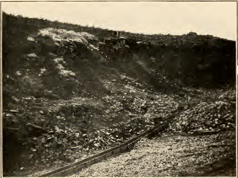
Fig. 2.--LOOKING UP FOX GULCH, BONANZA CREEK, NEAR DAWSON, CANADA Sluice box in the center, and the muck filling of the gulch not yet sluiced out may be seen in the background on the right
