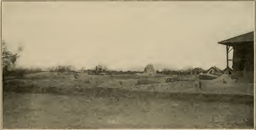
c View from outside north wall NORTHEAST BUILDING
