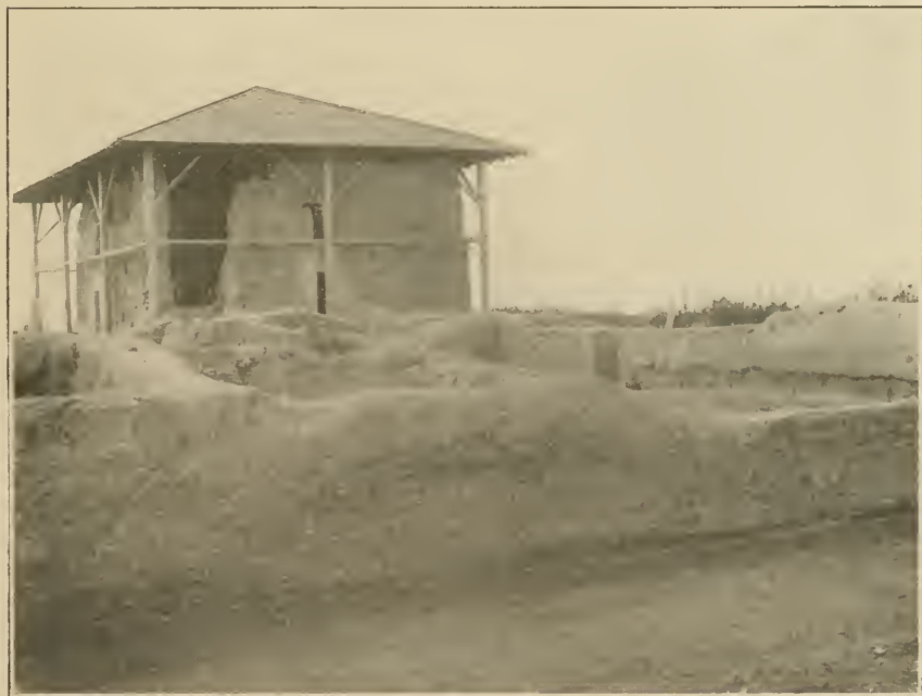
b View of north room from outside compound
