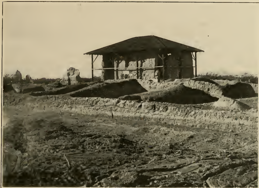
a View from outside east wall
