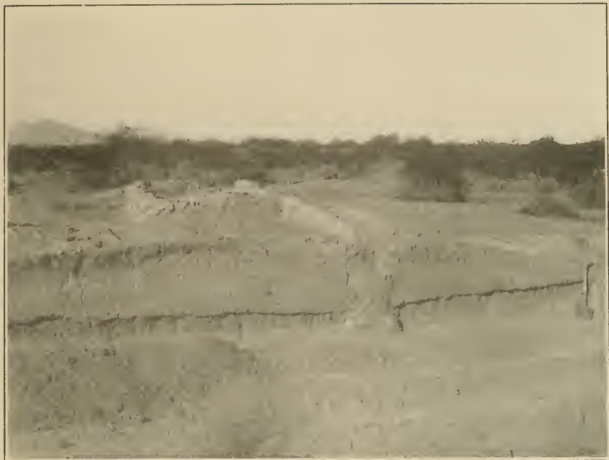
a View of east wall showing basal erosion
