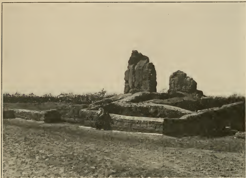
a View from northeast
