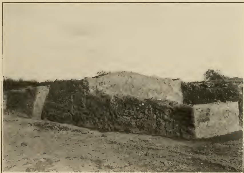
b View from northwest NORTHEAST BUILDING
