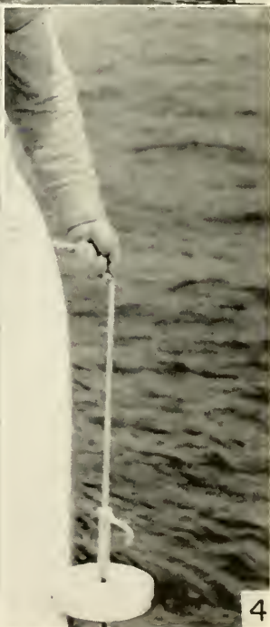
1, Hydroscope in use. 2, United States Navy hydrophotometer Mk II. 3, Specially designed hydroscope. 4, Secchi Disc.
