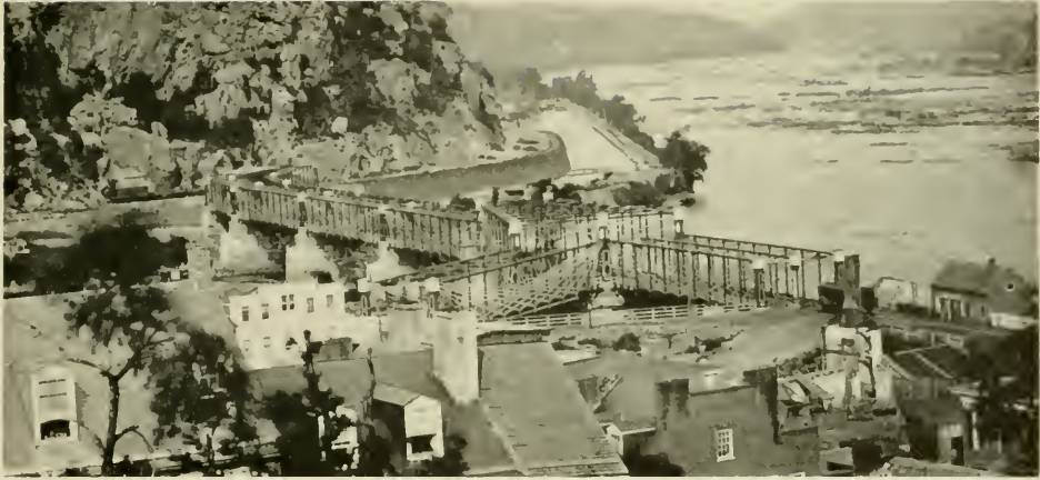
Figure 14.—THE HARPERS FERRY BRIDGE as completed after the Civil War. It was used by the Baltimore and Ohio until 1894, and as a highway bridge until 1936. (Photo 690, Baltimore and Ohio Collection, Museum of History and Technology.)
