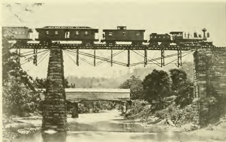
Figure 11.—THE FINK TRUSS. (Smithsonian photo 41436.)
