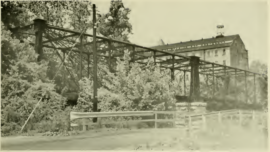
Figure 23.—THE ONLY SURVIVING BOLLMAN TRUSS BRIDGE, at Savage, Maryland. The bridge was built elsewhere in 1852 and was moved to this now-abandoned Baltimore and Ohio industrial siding in about 1888.
