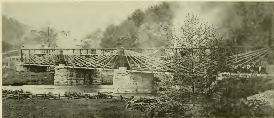
Figure 9.—BOLLMAN SKEW BRIDGE at Elysville (now Daniels), Maryland, built in 1853-1854. (Photo courtesy of Maryland Historical Society.)
