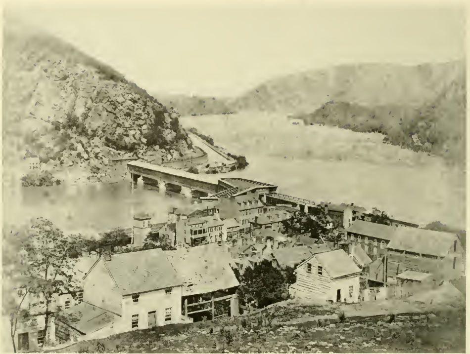
Figure 8.—THE BALTIMORE AND OHIO RAILROAD'S Potomac River crossing at Harpers Ferry, about 1860. Bollman's iron "Winchester span" of 1851 is seen at the right end of Latrobe's timber structure of 1836, which forms the body of the bridge. (Photo courtesy of Harpers Ferry National Historical Park.)
