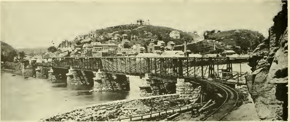
Figure 13.—THE FOUR BOLLMAN SPANS at Harpers Ferry that survived the Civil War. The spans were completed in 1862-1863. (Photo courtesy of Baltimore and Ohio Railroad.)
