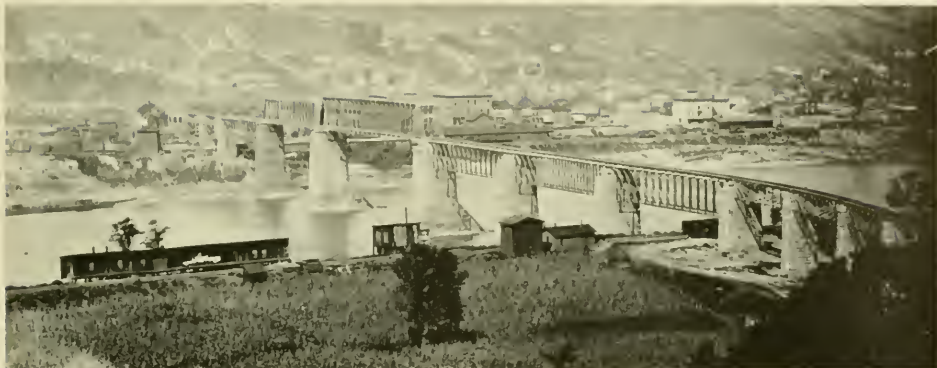
Figure 18.—OHIO RIVER CROSSING OF THE BALTIMORE AND OHIO AT BENWOOD, West Virginia, completed in 1870. Bollman deck trusses were used in the approaches on both sides. (Photo 693, Baltimore and Ohio Collection, Museum of History and Technology.)
