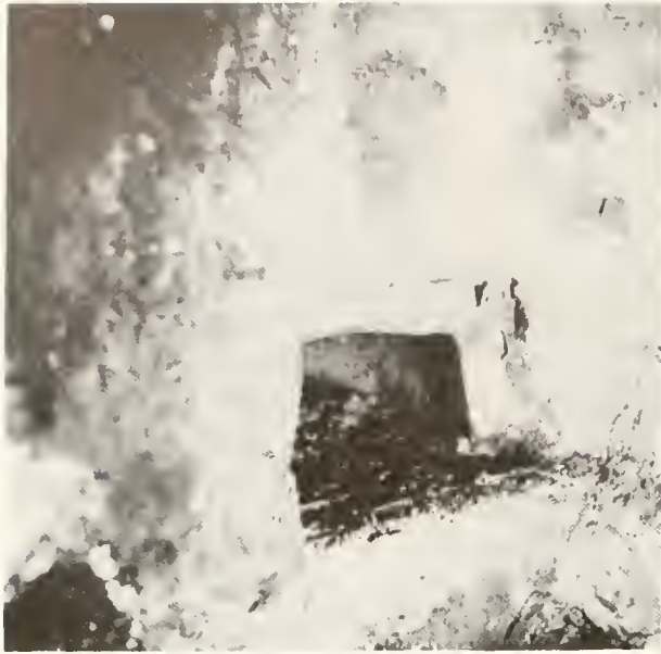
FIGURE 8.—Views of opening of oven in figure 7, photographed before its removal from house. This illustrates how oven was built into corner of fireplace and concealed from view. At right, the oven door is in place. (Photos by A. C. Littlejohns.)
