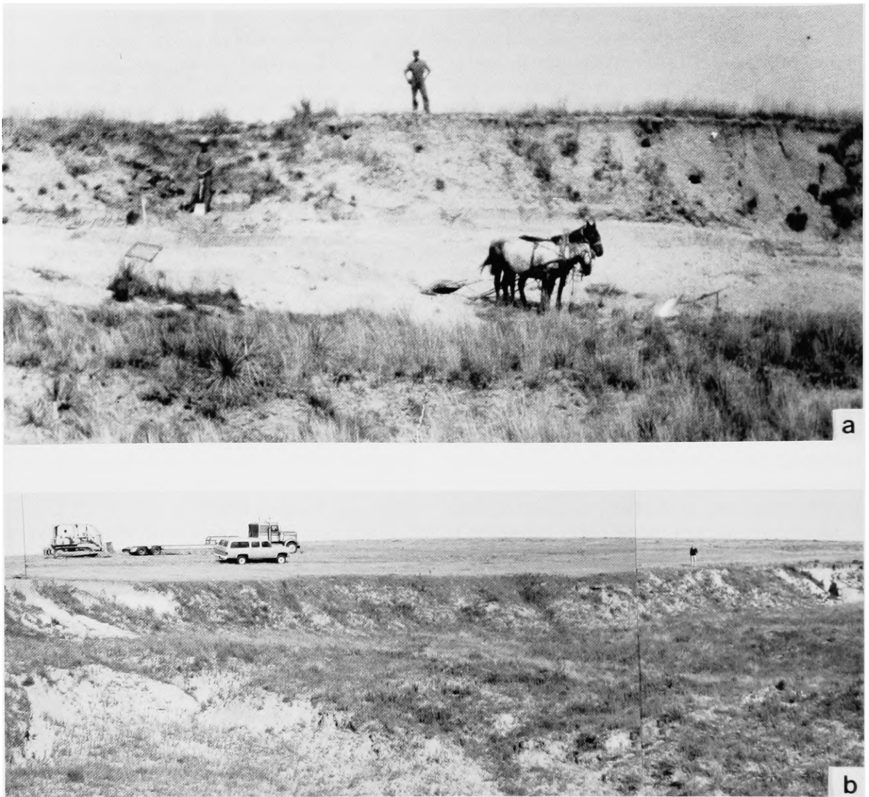
FIGURE 2.— a , Edson Quarry in late 1920's during excavation by H.T. Martin and C.J. Hesse; b , Edson Quarry in 1977.
