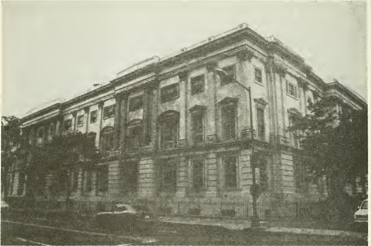
Exterior view of the General Post Office Building at 7th and G Streets, N.W. (Photo by Jeff Ploskonka)
