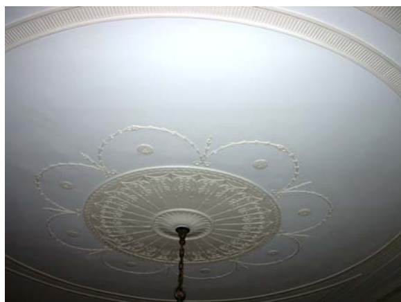
Figure 66. Blair Library Ceiling
