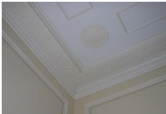
Figure 67. Blair Library ceiling corner
