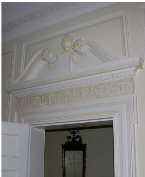
Figure 65. Blair Library door detail with broken pediment, rosette and urn motif trims
