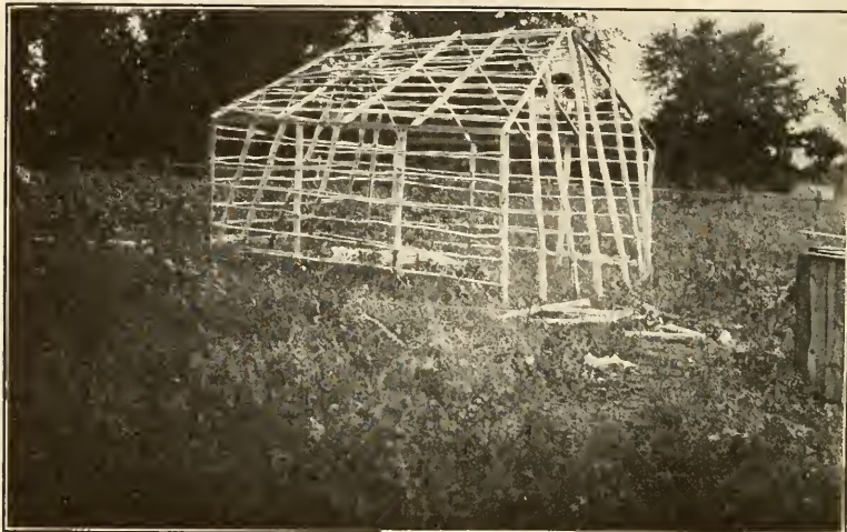
a , Frame of structure to be used for mat weaving
