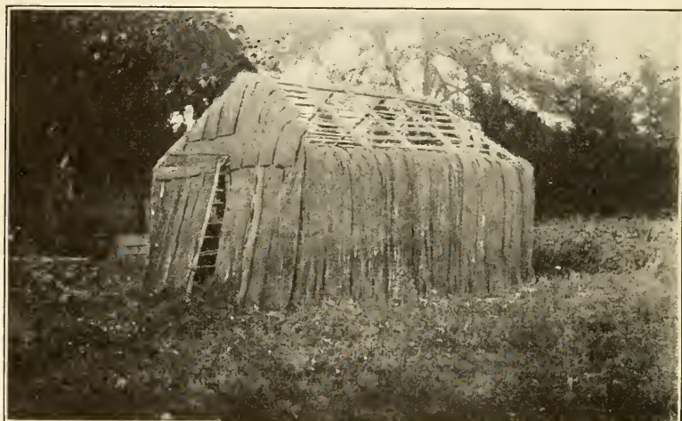
b , Partially completed structure to be used for weaving
