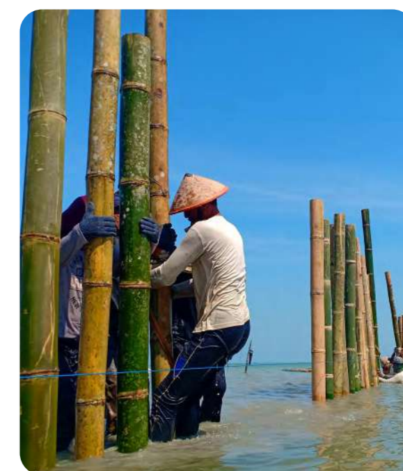
Community members work together to construct a permeable sediment trapping structure in Timbulsloko Village, Indonesia. © Kuswantoro
