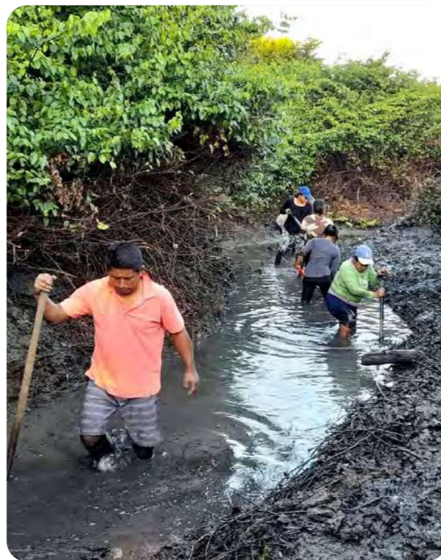
Dredging channels on mangrove sites in Barra de Santiago. © IUCN / USAID
