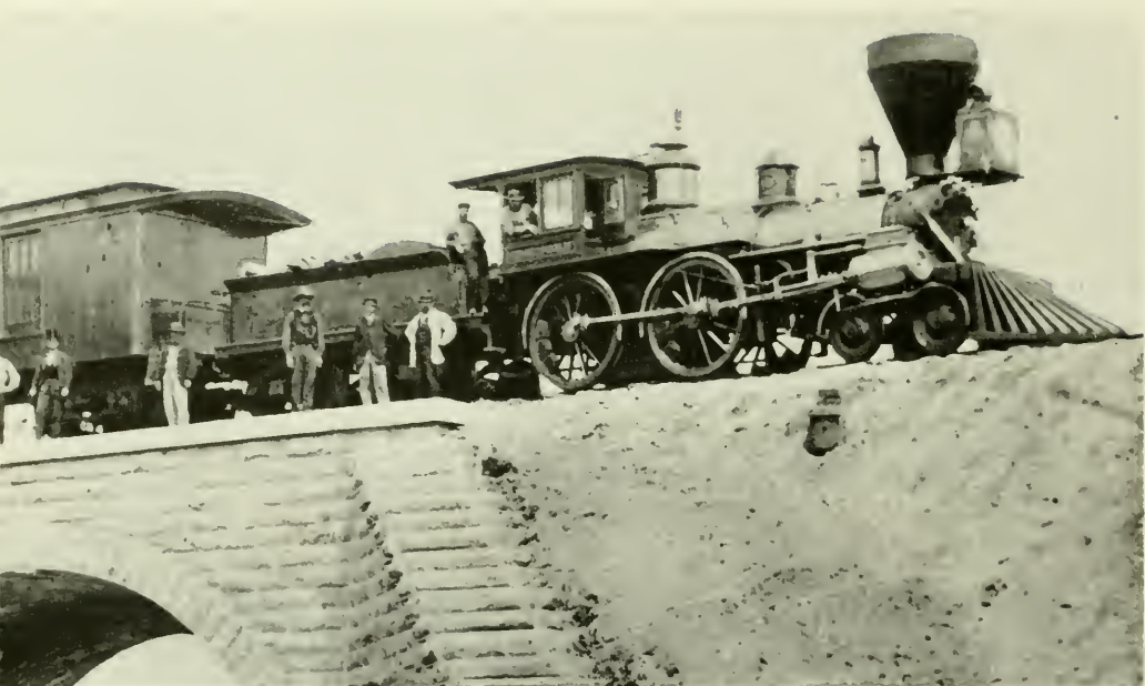
Figure 51.—THE “ELKHORN” OF THE CHICAGO AND NORTHWESTERN RAILROAD, built by Niles in 1858. Scene is Askew Arch Culvert, near Rockford, Ill. (Photo courtesy A. W. Johnson.)
