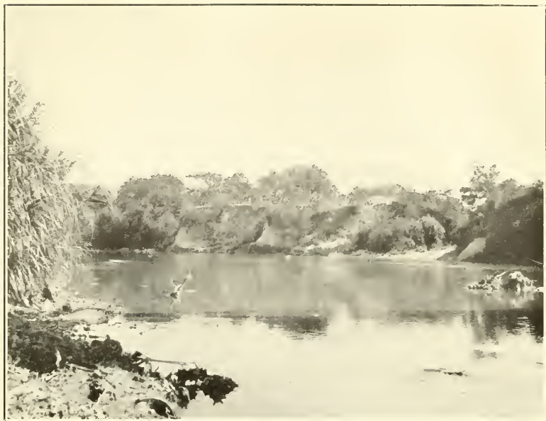
ARTIBONITE RIVER NEAR LAS CAHOBES, HAITI
