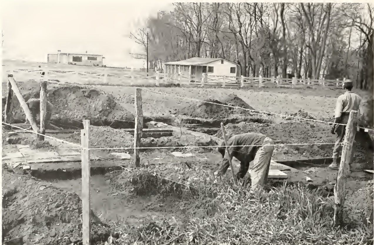
Figure 47.—FOUNDATION of Structure E (kitchen).
