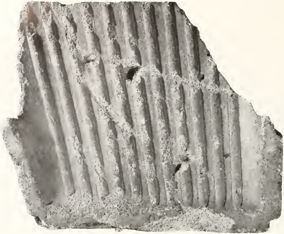
Figure 40. CAST-CONCRETE BLOCK, probably part of a rusticated door en- framing. Found at south end of Structure B. (See ills. 1 and 2.)
