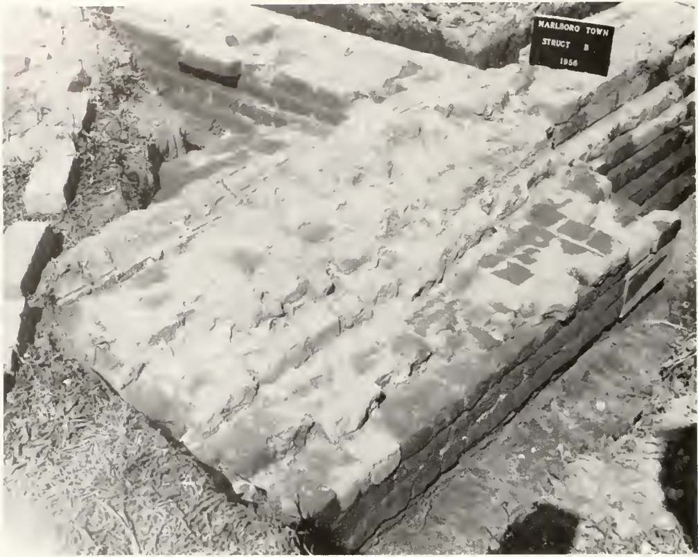
Figure 35.—SOUTHWEST CORNER OF STRUCTURE B, showing molded-sandstone trim with added brickwork in front. Bricks also covered red-sandstone block, lower right. (Diagonally placed bricks at left are not part of structure.)
