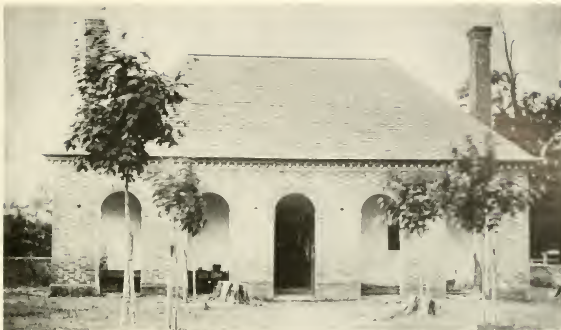
Figure 5. KING WILLIAM COURTHOUSE, about 1725. Mercer often pleaded cases here. (From a Civil War period negative. (Courtesy of Historic American Buildings Survey, Library of Congress. )
