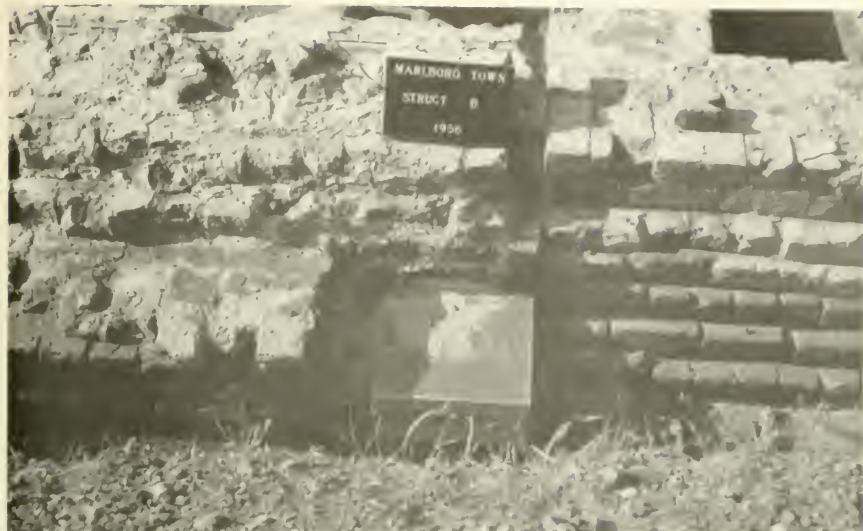
Figure 34. SOUTHWEST CORNER OF STRUCTURE B Piazza foundation extended south with red sandstone block at junction of piazza with main foundation. To the left of top of sign, molded red-sandstone trim can be seen which apparently surrounded the piazza. Bricks in front of trim appear to have been added later as a platform. Brick foundation of main-foundation footing appears at right.
