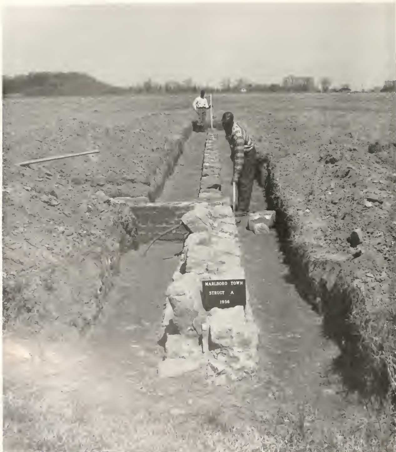
Figure 25. — Looking north in line with Walls A and A II. Wall A I joining at right angles.
