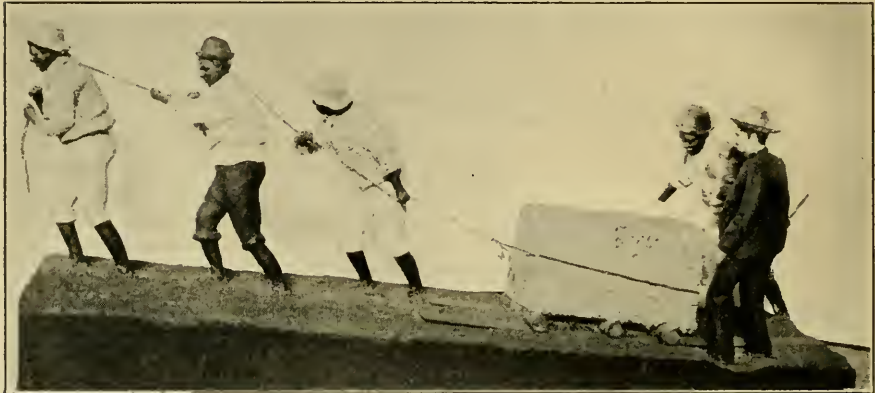
FIG. 1.—THE COMBINED APPLICATION OF THE ROLLER, LEVER, AND INCLINED PLANE.
